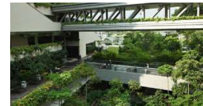
05. CETRAM (Hospital-Parque) Hospital Khoot Tek Puat, Singapur
