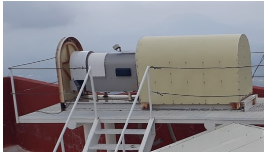
Fig. 1.8: RPG-Tip-225 radiometer installed at the roof of the LMT's Visitor Center building.
