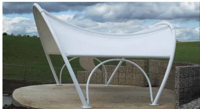
Fig. 15: Pabellón Campbell park, vista lateral
