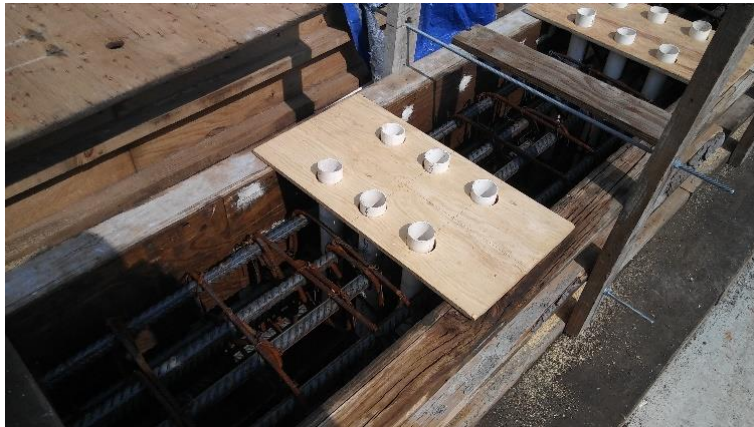
Figure 6-7. PVC pipes in the column formwork.
