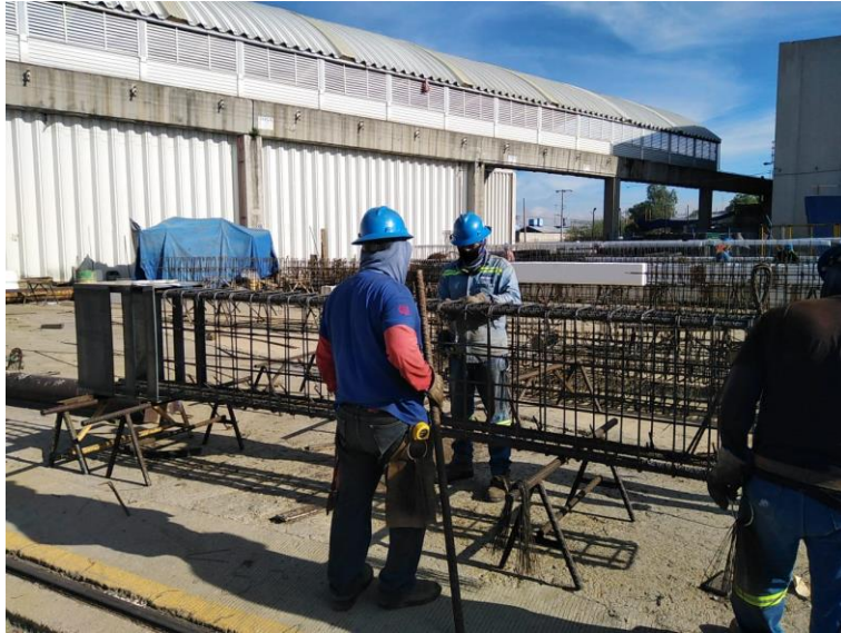
Figure 6-49. Beam assembly.
