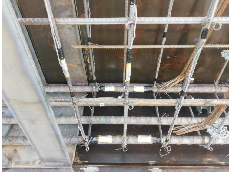
Figure 6-51. Strain gauges on longitudinal and transverse reinforcement.
