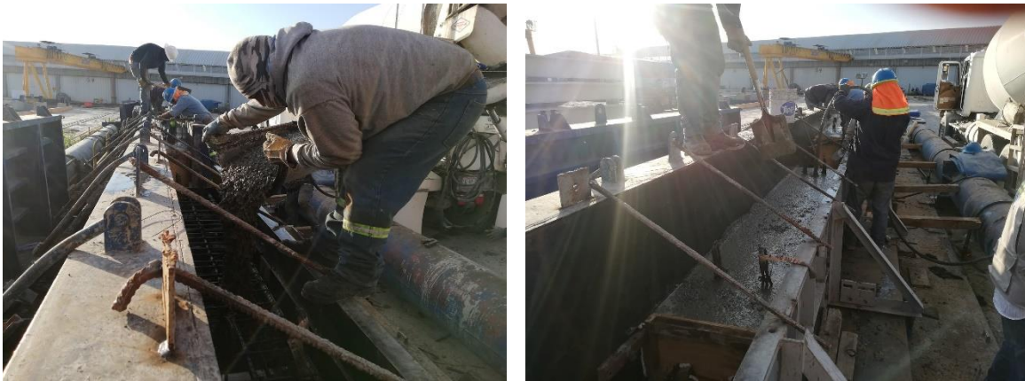
Figure 6-54. Casting of the column.
