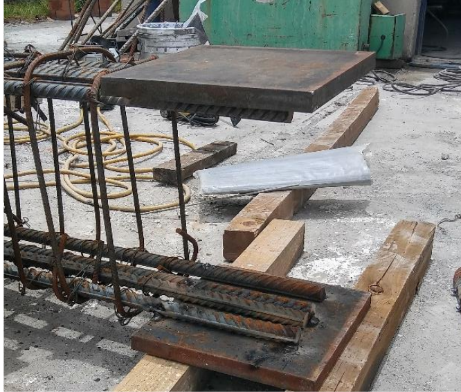
Figure 6-6. Welding of reinforcing steel to the steel box.
