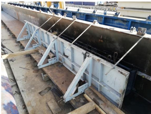
b) Formwork securing
