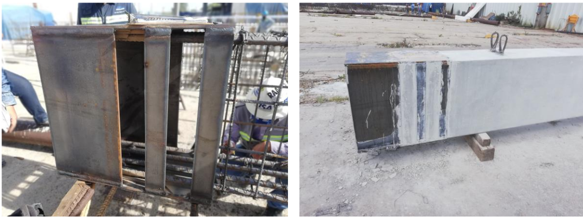
a) Before concrete pouring
