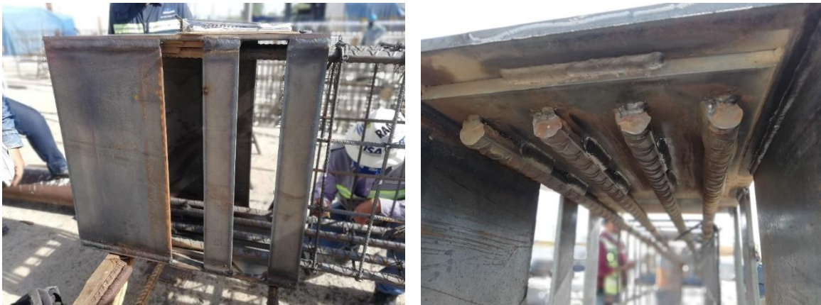
Figure 6-50. Steel box and welded rebars.
