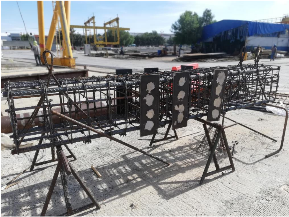
a) Before pouring of concrete
