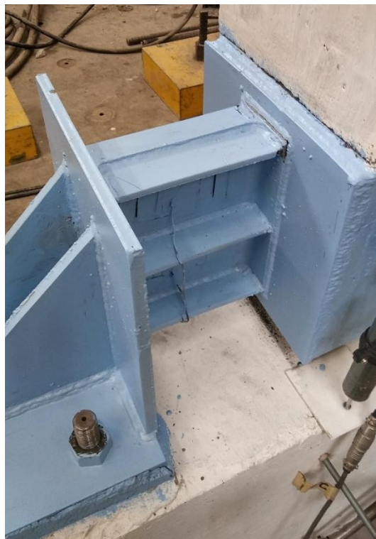
Figure 5-20. Weld failure at beam-damper interface.
