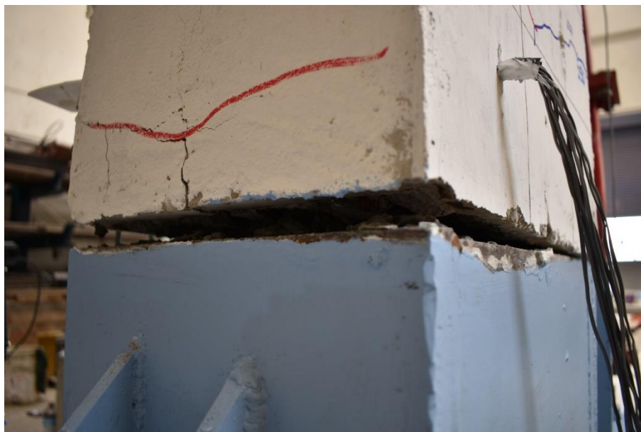
Figure 5-21. Simultaneous fracture of beam rebars of specimen P-ID-1M.
