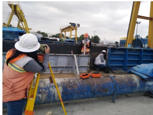
a) Placement of formwork
