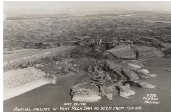
Figura 2.1 Falla de flujo de la Presa Fort Peck, Montana, EE.UU. (1938). (Association of state dams safety, 1984)
