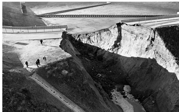
Figura 2.3 Falla de Presa Balwin en California, EE.UU. (1963). (Association of state dams safety, 1984)
