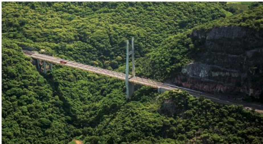
Figura 2.20. Puente Barranca El Zapote (SICT, 2015)
