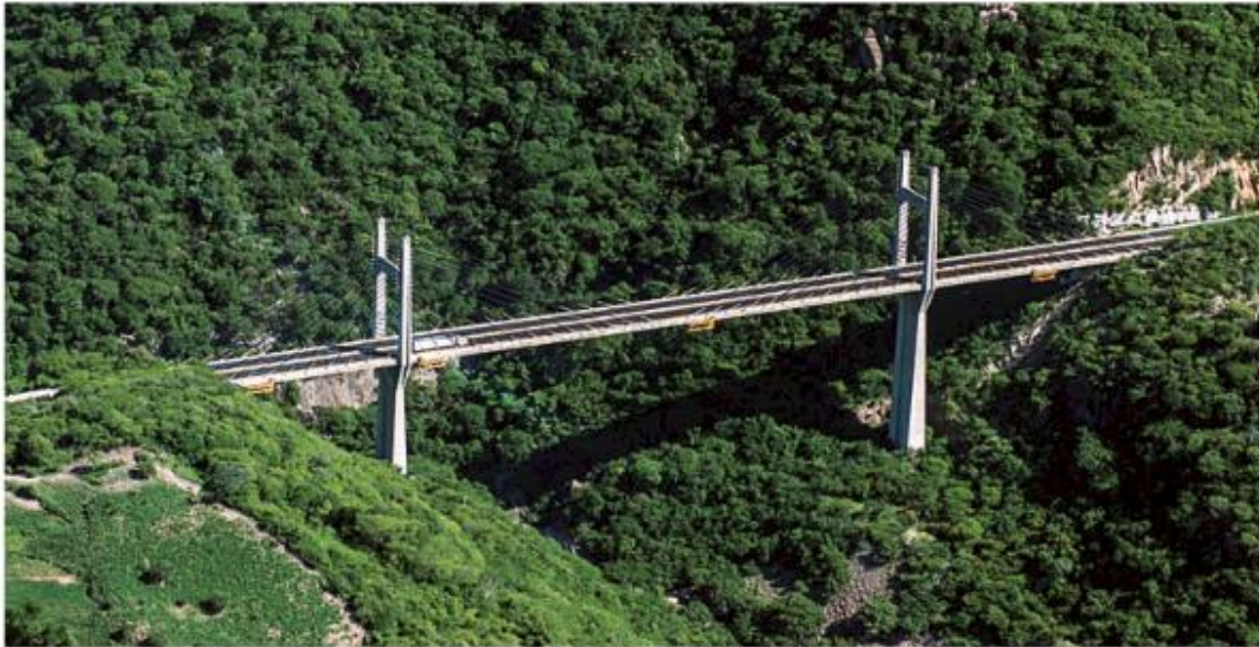
Figura 2.18. Puente Quetzalapa (SICT, 2015)
