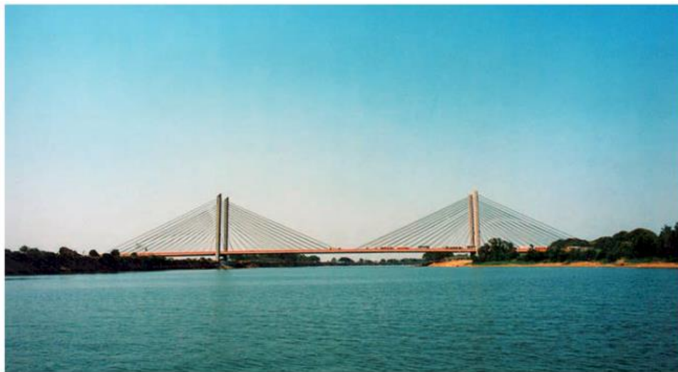
Figura 2.24. Puente Papaloapan (SICT, 2015)
