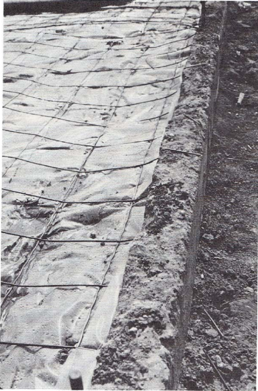
Figure 9.10 Mesh installation.
