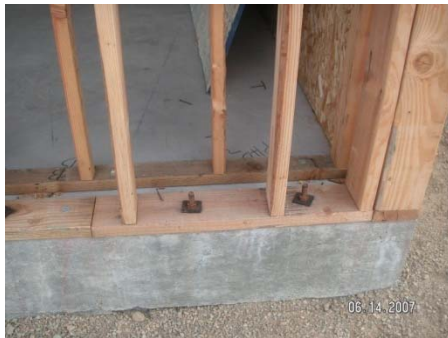
Fig. 8-21. Nonbearing partitions.
