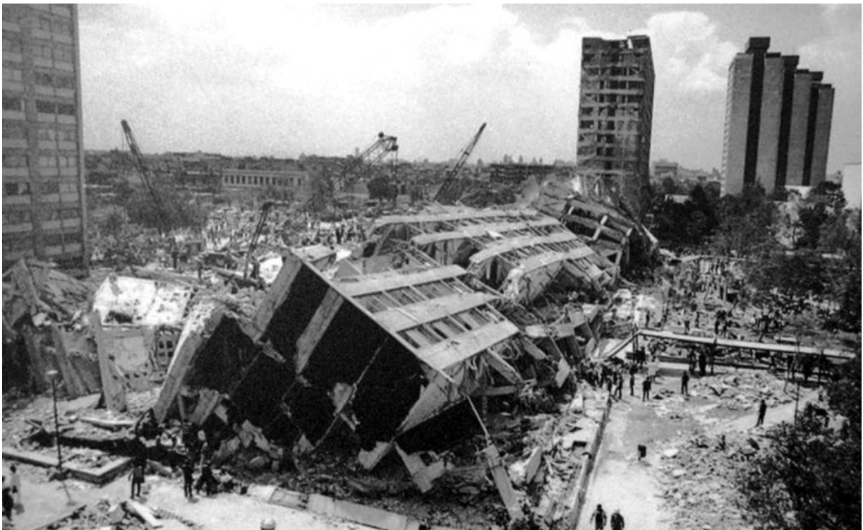
Figure 1.1 Total collapse of a 15-story reinforced concrete building located in Tlatelolco, Mexico City due to the September 19, 1985 earthquake. The photograph was taken from the El Universal newspaper archive 21
