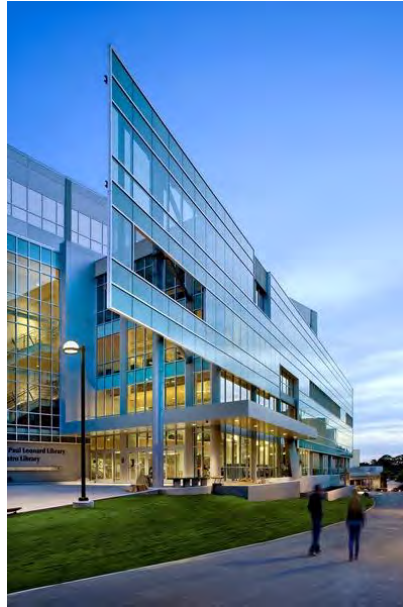
1.3.4. San Francisco State University, J. Paul Leonard and Sutro Library (fotografía de David Wakely tomada de Internet, HMC Architects )
