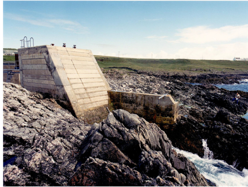
Figure 3.3: Shoreline OWC device on the island of Islay, Scotland (Falcão and Henriques; 2016).
