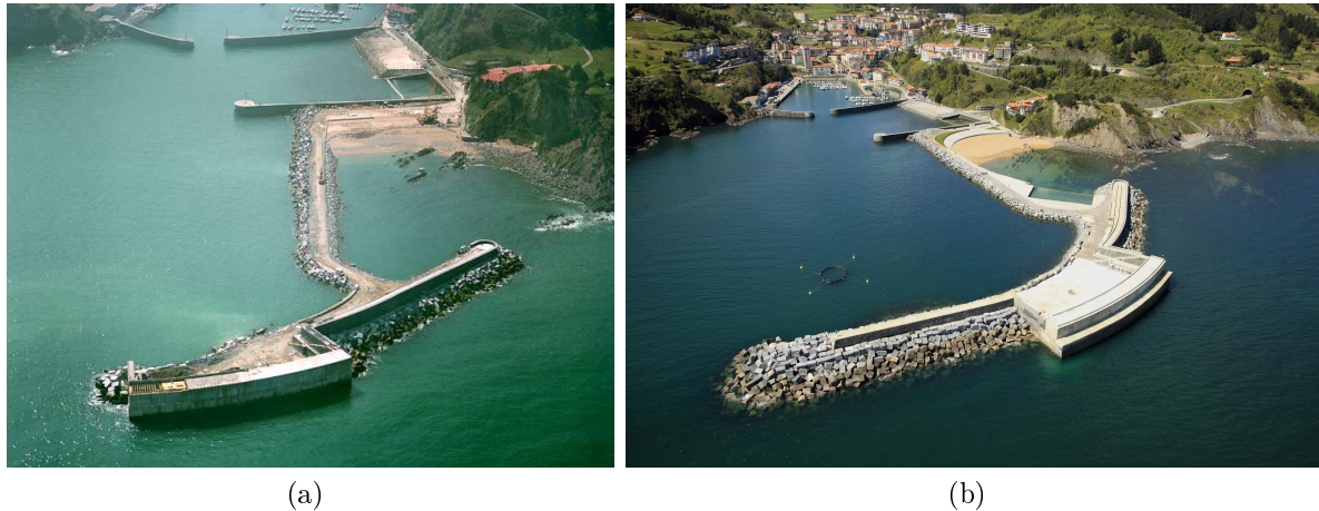
Figure 5.2: Comparison between the original and the present-day design of the integrated breakwater-OWC system in Mutriku. (a) View of the MWEP in 2008 (Reproduced with permission from Torre-Enciso et al. (2009)). (b) Mutriku OWC (source: EVE ( Ente Vasco de la Energía ; n.d.)).
