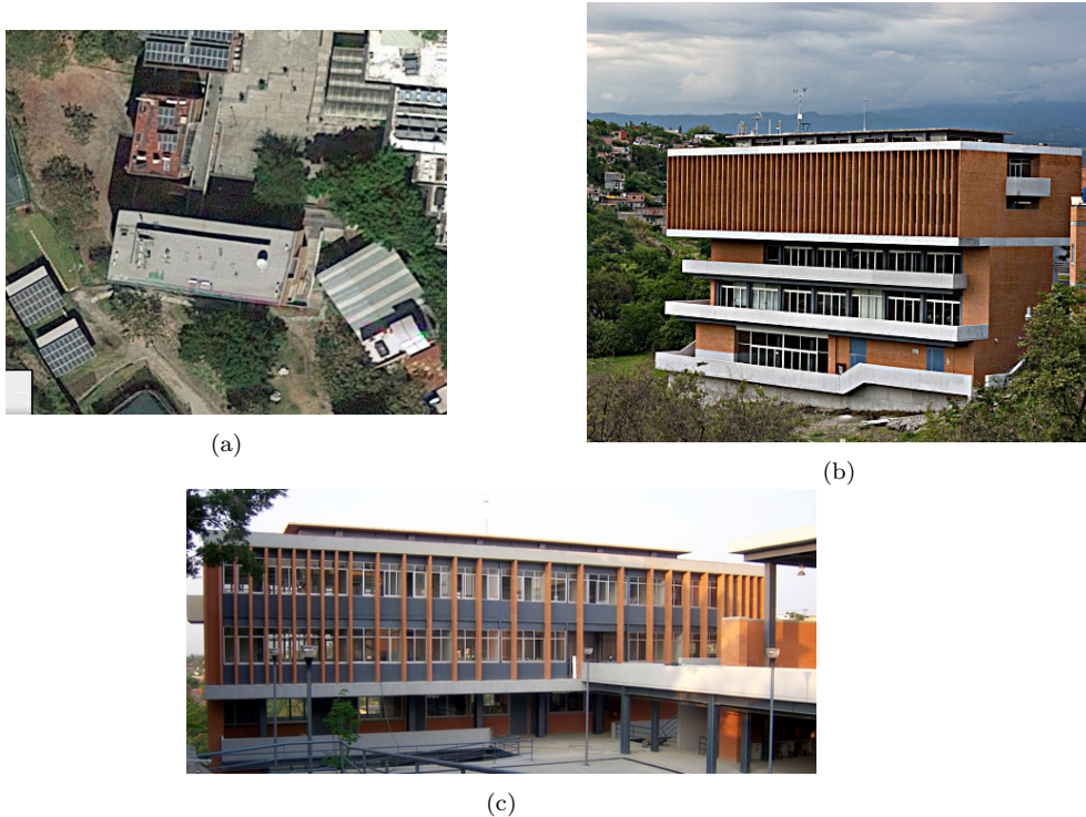
Figure 1: Views of the building. (a) Aerial view, (b) view of the South façade and (c) view of the North façade.
