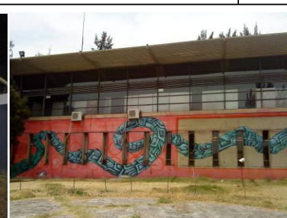
NAVE PRINCIPAL - GALERIA
