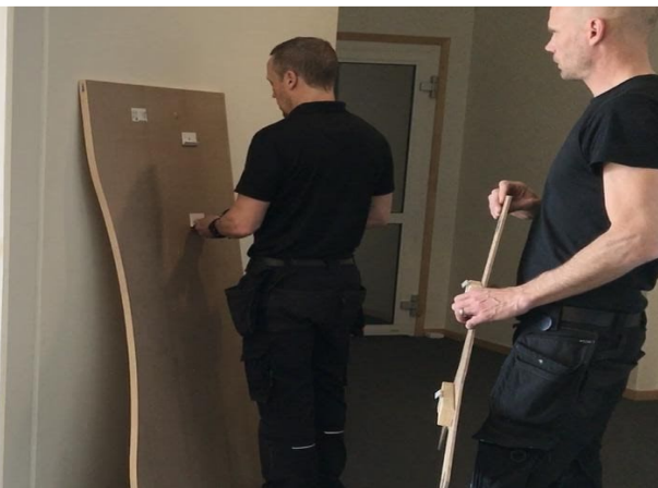
Figure 74. Mounting test hangers-system.
