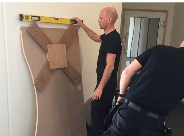
Figure 75. Mounting test two holes-system.
