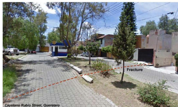
Figure 1. Photo of Querétaro, Cayetano Rubio Street, showing the effect of differential land subsidence due to groundwater withdrawals. The large displacement gradients are responsible for earth fissuring producing significant economic losses and increasing the safety issues in the urban area.
