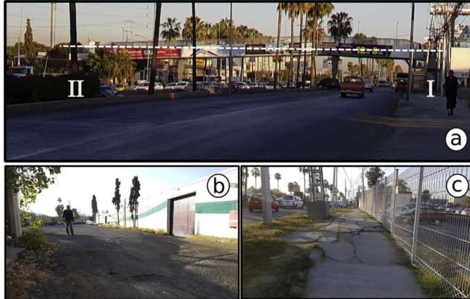
Fig. 1. Photographs showing some of the effects of differential land subsidence due to groundwater withdrawals in Querétaro: a) panoramic view of the 5 de Febrero Avenue (looking North), with the ground fracture displacements that have affected both the street and the bridge built originally horizontal between I and II; b) ground fractures have produced differential vertical displacements larger than 1.5 m; c) recent displacements (2016–2017) on 5 de Febrero avenue (looking south) along the trace of the Central Fault. The photographs were taken in the highest subsidence area defined by Chaussard et al. (2014).
