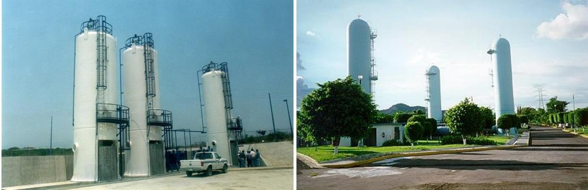
FIGURA 4.5-15 CÁMARA DE AIRE INSTALADAS EN UN ACUEDUCTO EN LINARES-MONTERREY (IZQ.) Y CHAPALA-GUADALAJARA (DER.).
