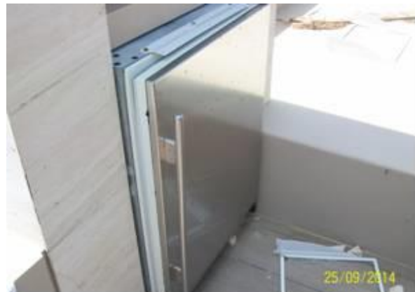
Outdoor kitchen with corrosion stains. Steel refrigerator with corrosion stains (roof).
