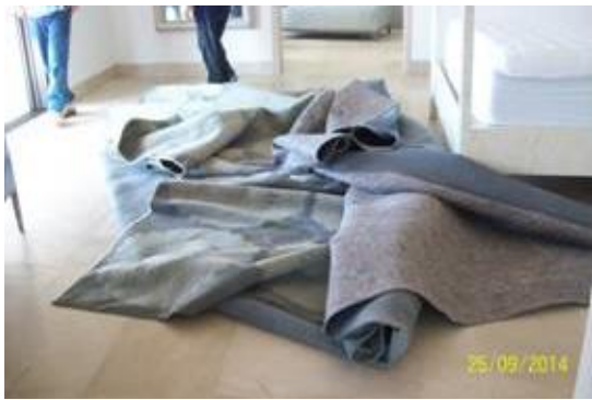
Rugs and carpets with water damage
