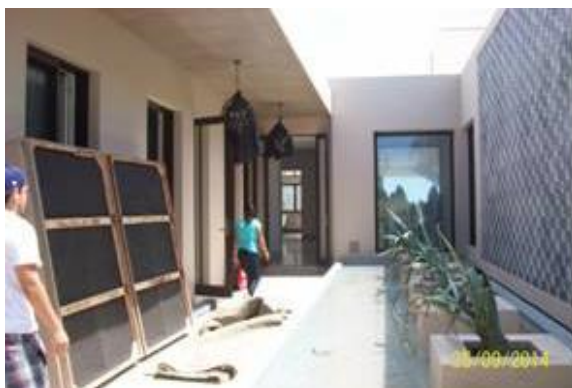
Outdoor corridor - entrances to bedrooms
