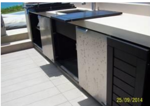
Outdoor kitchen with corrosion stains. Steel refrigerator with corrosion stains (roof).
