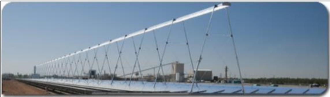
Imagen 2.11. Reflector lineal Fresnel. [Areva solar, 2012]
