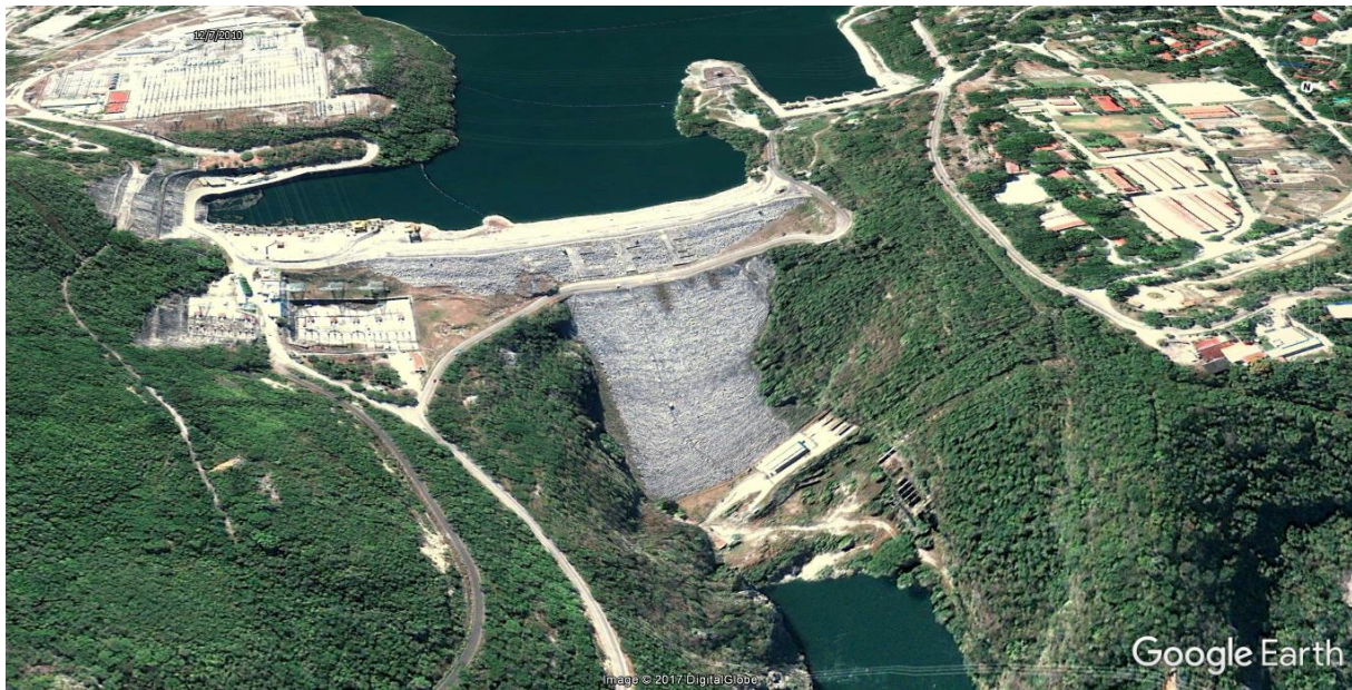
Figura 3.9. Presa Ing. Manuel Moreno Torres (Google Earth)
