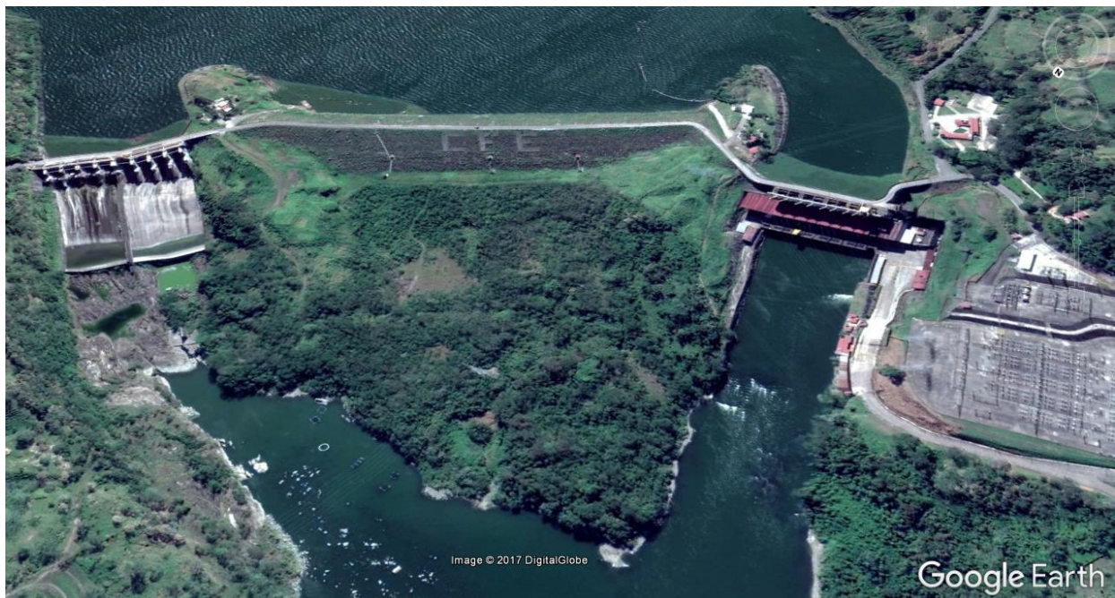
Figura 3.13. Presa Peñitas (Google Earth)
