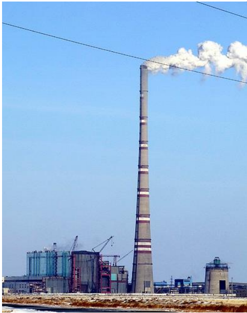
"Gres-2 Power Station"
