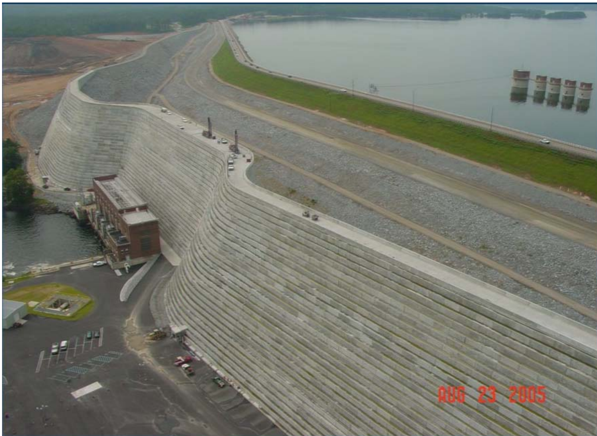
Figura 1- 27 Saluda Dam Rehabilitada (Rizzo C., 2008)
