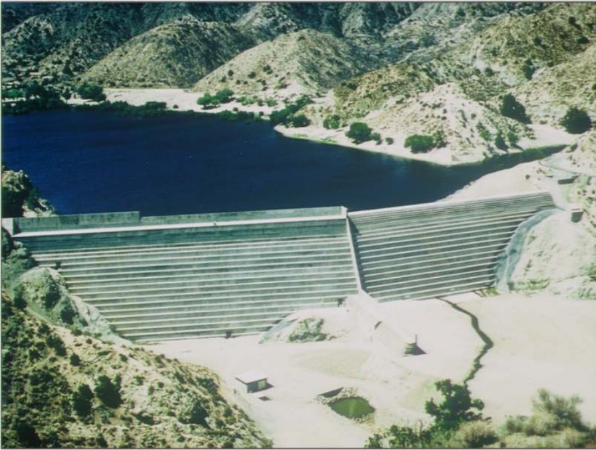
Figura 1- 24 Littlerock Dam California Rehabilitada con CCR (Hansen K. , Rehabilitation of Existing Dams with RCC, 2008)
