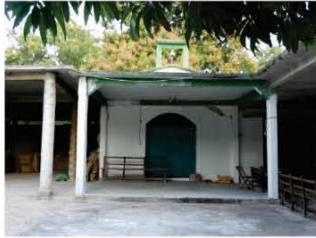
FACHADA PRINCIPAL CAPILLA MAYOR
