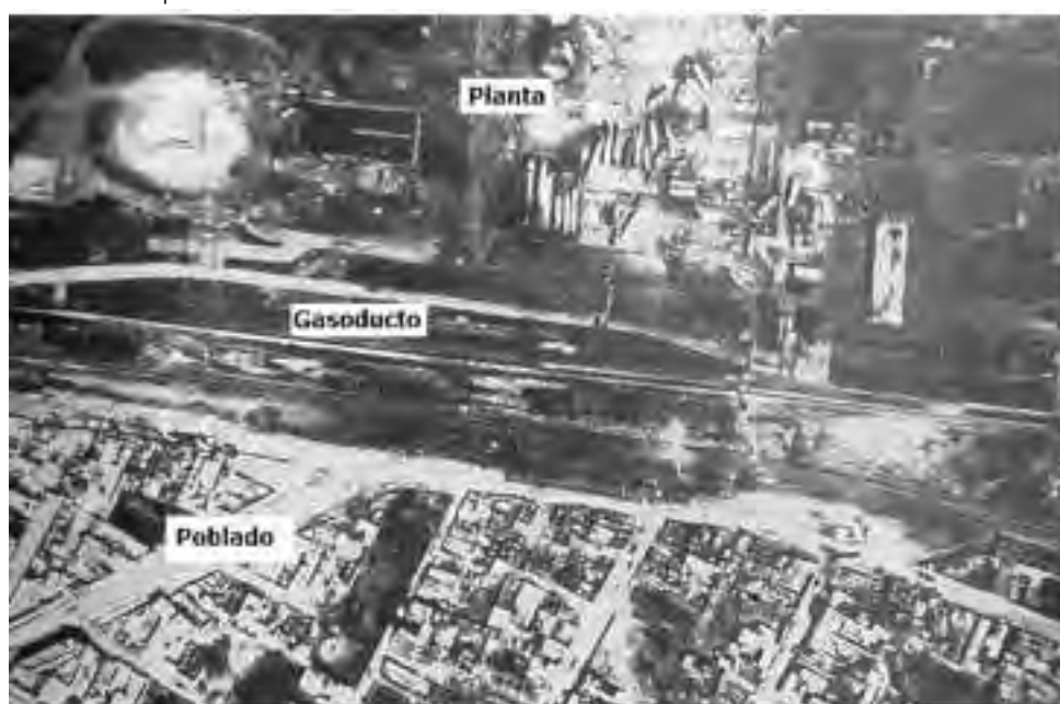
Figura 5.10 Planta de almacenamiento de Gas LP. San Juan Ixhuatepec. Fuente ( http://www.unizar.es/guiar/1/Accident/San_Juan.htm ) [62].
