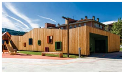
Vista 2. Fachada interior
