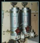
Solid Fuel Oxygen Generator (SFOG), burns candles to produce oxygen as a backup system.
