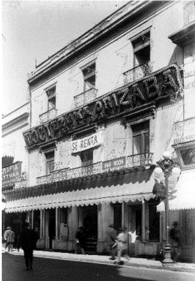
Figura 2. Restaurant-bar Bach, fachada.
