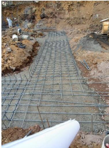
Fig. 6.8 “Zapata corrida armada”
