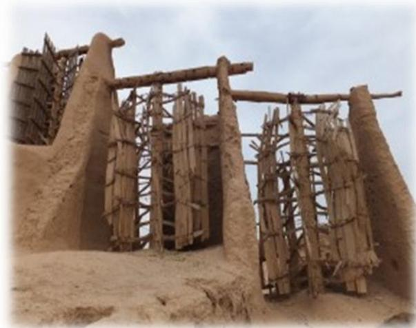
**Figura 2. Molino de viento persa. Fuente: [www.renewableenergyworld.com](http://www.renewableenergyworld.com)**
