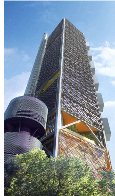
Torre Bancomer 225 m
