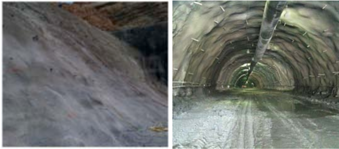
Figura 1.1 Túnel Grijalva, Chiapas, México, shotcrete fibras Dramix RC65/35BN (Bekaert)
