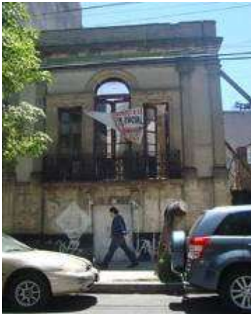
Fachada principal, predio Sabino No.89
