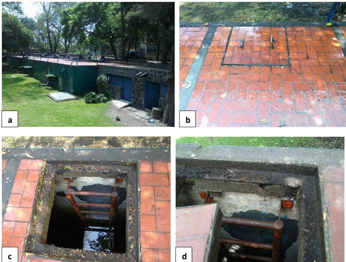
Figura 1 a, b, c, d. Cisterna Campus Central
