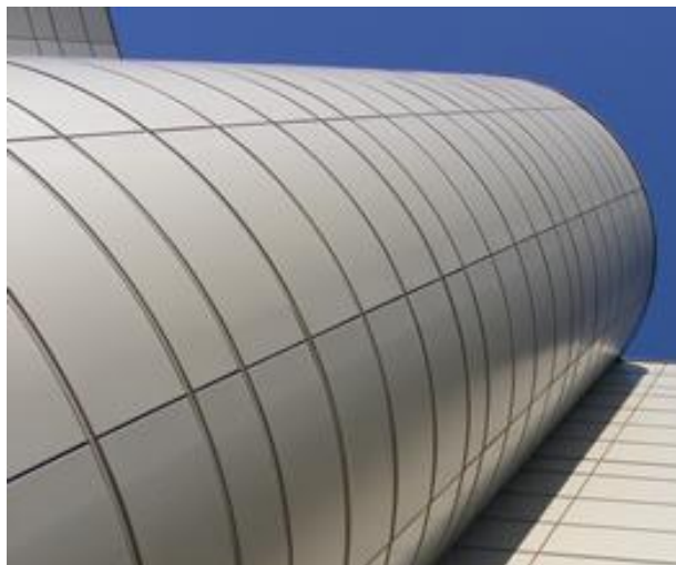
Paneles curvos de Alucobond.
