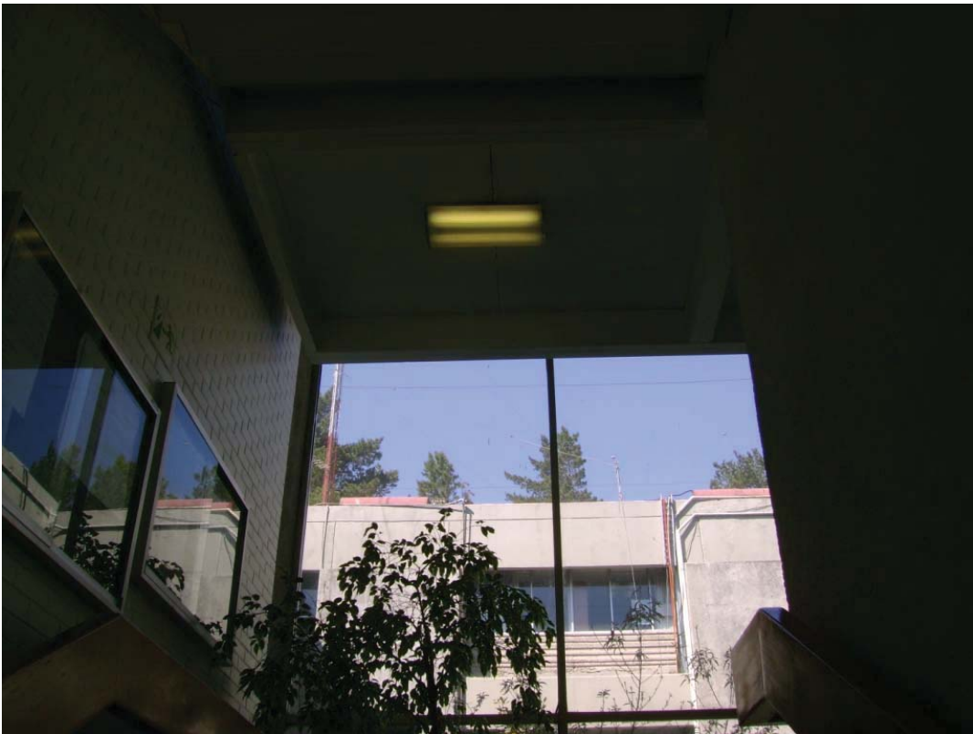
Escaleras PB-1N (10:44hrs)
