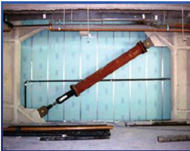
Figura 4.1: Amortiguador Viscoso (VD). (Copyright © 2012 Taylor Devices All Rights Reserved)
