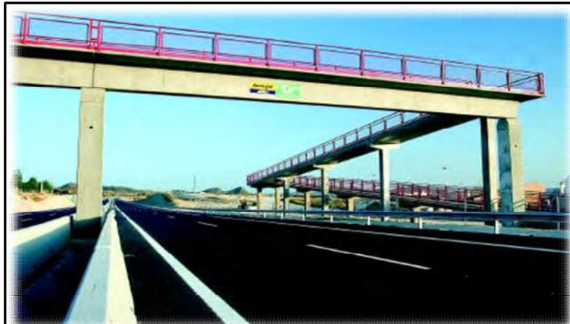
FIG. 16 PASO INFERIOR PEATONAL (P.I.P) CON RAMPAS LATERALES.
