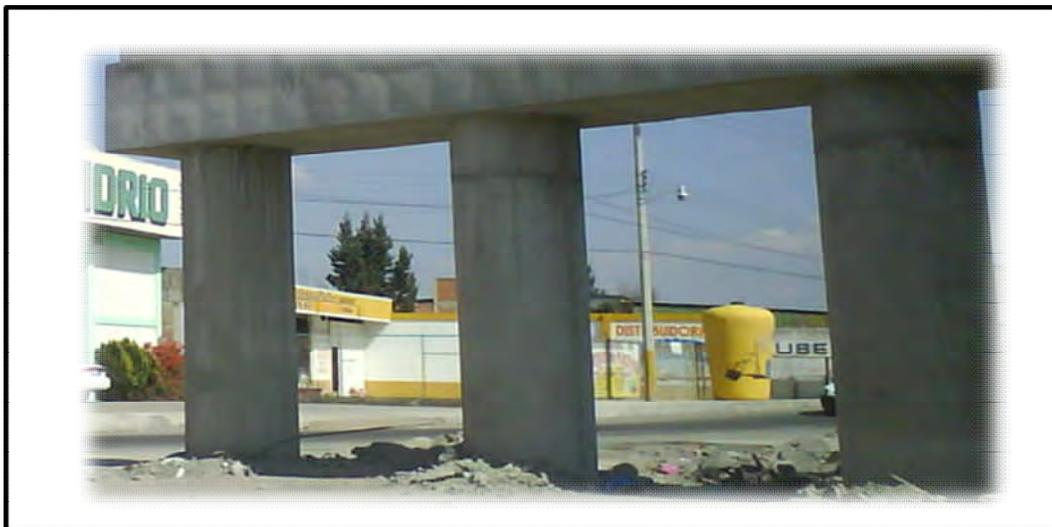
FIG. 27 SISTEMA DE PILA TIPO COLUMNA, EN DONDE SE MUESTRA EN SU PARTE SUPERIOR AL CABEZAL.
