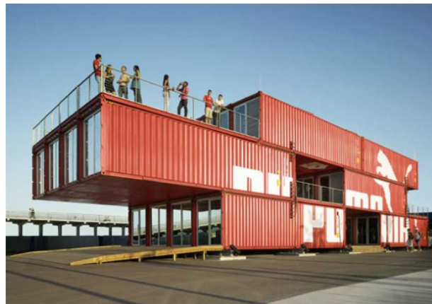
FIGURA 13. Container Mall. Lot-EK
