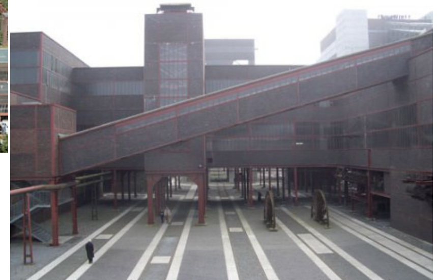
Fachada Interior. http://urbanigloos.wordpress.com/category/sustainability/
