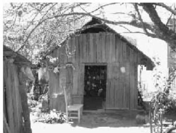
Figure 3. Kitchen structure with ventilation between the walls and roof.
