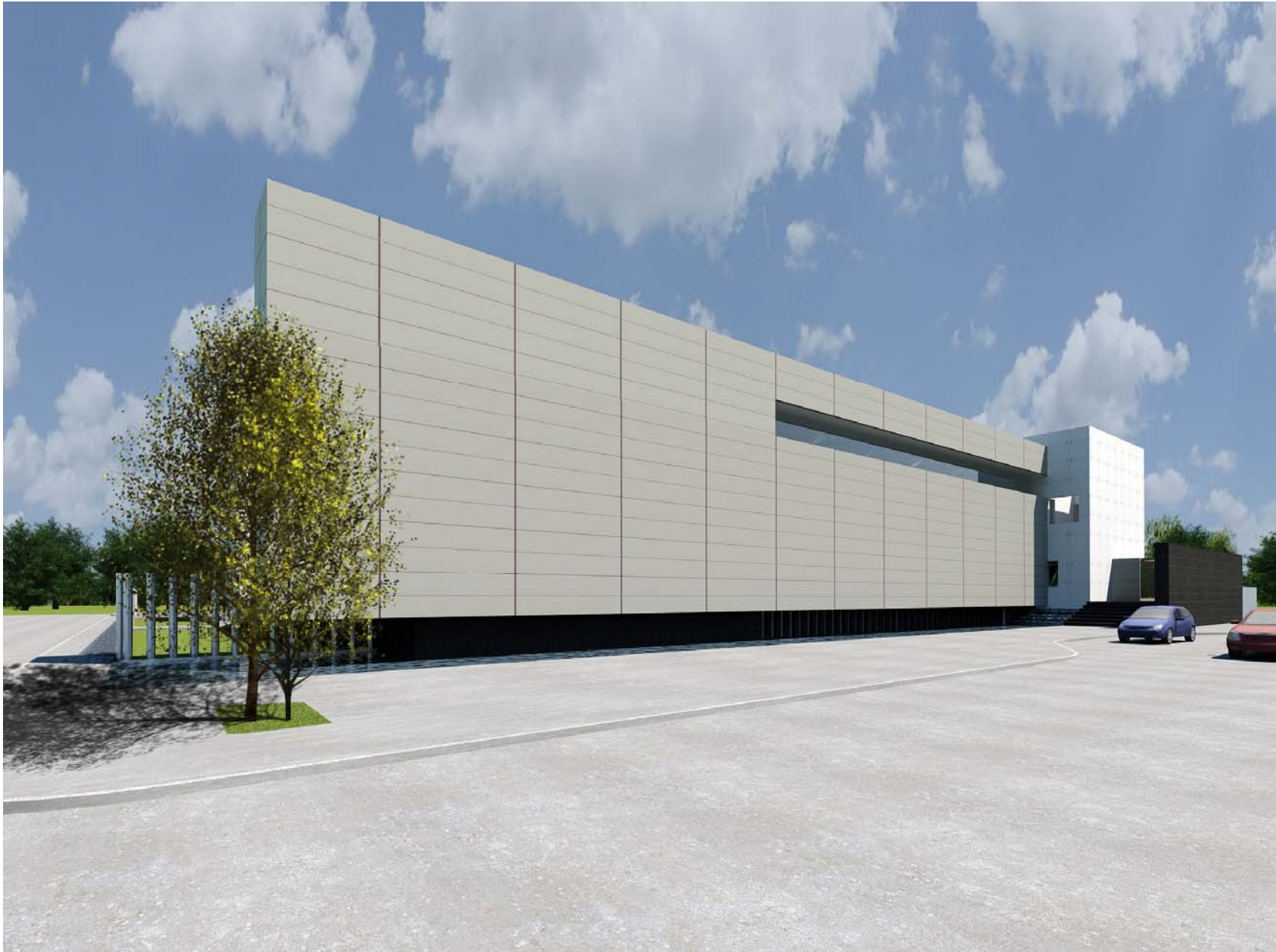
FACHADA PRINCIPAL (NORTE)
