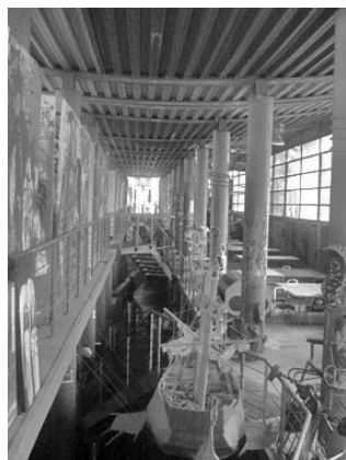
Talleres 2 Nave Principal y Pasillo Principal
