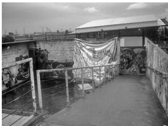
Salida Nave Industrial
