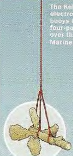
4,750-pound propeller and shaft were hoisted by the Kellie Chouest's forward crane.
