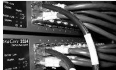
**Figura 1.9** Conector RJ45 en switch Ethernet.
