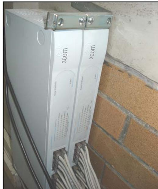
FOTOS 4.18 Y 4.19 SWITCHES 2X24 PARA EL LABORATORIO 2
