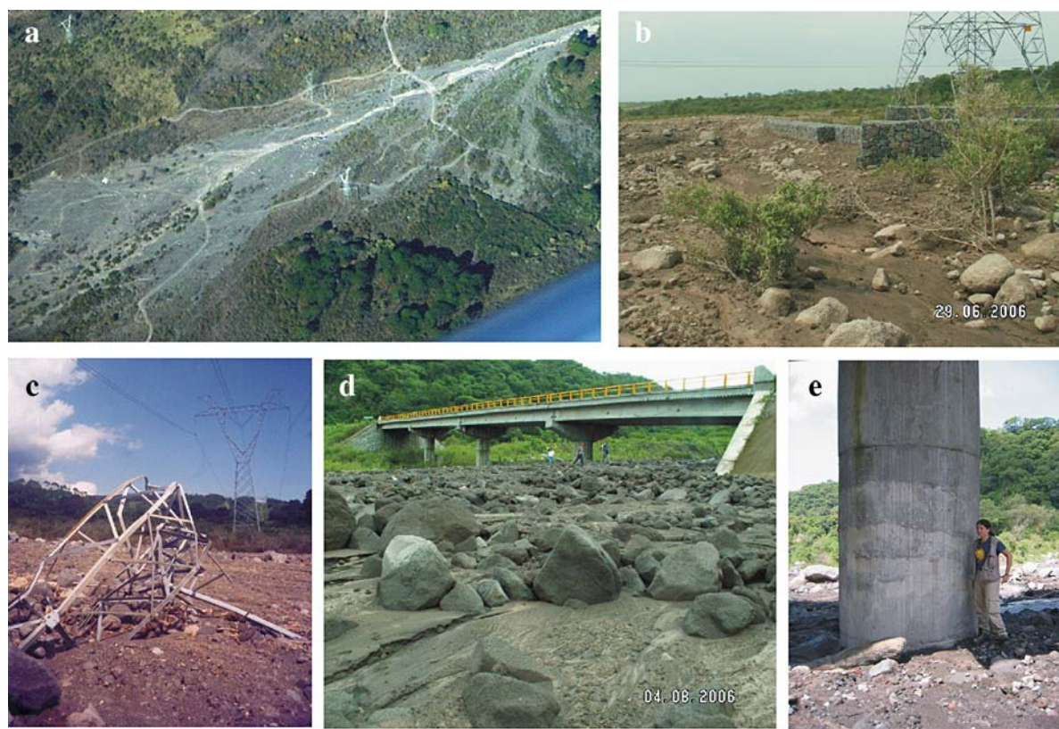
Fig. 4. Photos showing the several examples of damages provoked by lahars. a, b and c) Aerial view of the 1999 lahar in the Montegrande ravine where electric lines have been destroyed, note that the electric lines are now protected by a small rock barrier. d and e) Bridge over La Lumbre ravine where lahars charged with metric-sized blocks partially damaged the structure.
