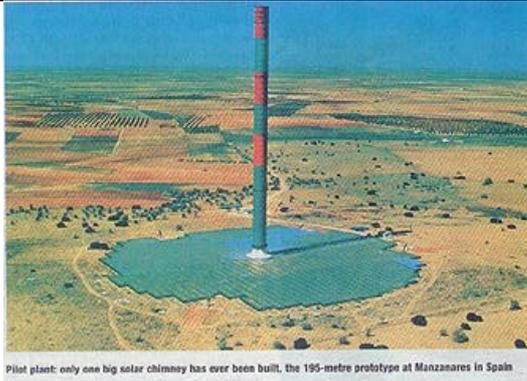
Pilot plant: only one big solar chimney has ever been built, the 195-metre prototype at Manzanares in Spain
