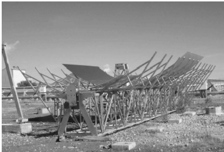
Figura 1.6. Estructura de soporte del Eurotrough. Fuente: Esteban, Osuna, Zarza, Nava. CIEMAT-PSA y Flabeg Solar Internacional, "Eurotrough design issues and prototype testing at PSA", Proceedings of Solar Forum 2001, Solar Energy: The Power to Choose, April 21-25, 2001, Washington, DC.
