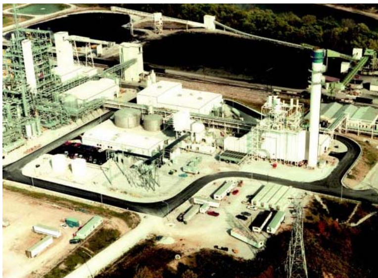
Fig. 1.3 Central CCGI de Wabash River, Indiana, EU. (Fuente: “ The Wabash River Coal Gasification Repowering Project ”)
