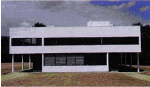
Villa Savoye. Fachada frontal.
