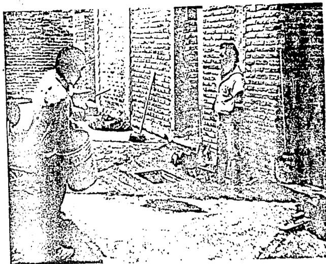
COLADO DEL PATIO DE LA VECINDAD, CON CONCRETO  $f'c= 120 \text{ Kg/cm}^2$  ARMADO CON MALLA ELECTROSOLDADA,  $e=8 \text{ cms.}$  Y COLOR ROJO OXIDO INTEGRAL.
