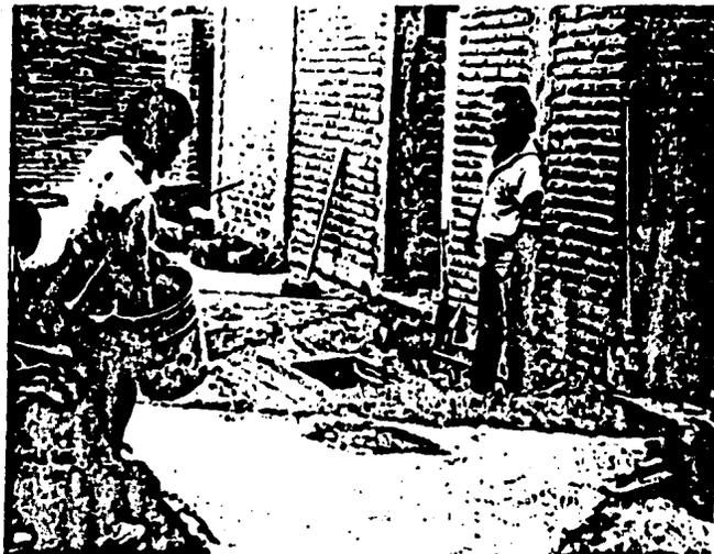
COLADO DEL PATIO DE LA VECINDAD, CON CONCRETO  $f'c= 120 \text{ kg/cm}^2$  ARMADO CON MALLA ELECTROSOLDADA,  $e=8 \text{ cms.}$  Y COLOR ROJO OXIDO INTEGRAL.
